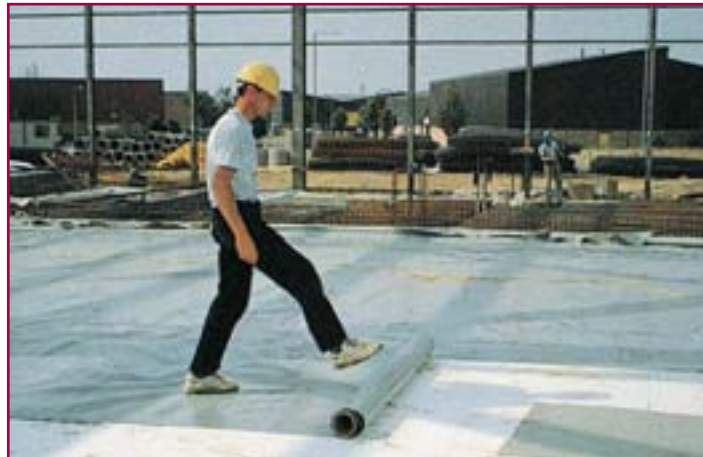
The use of Ventform with its sympathetic surfaces enables the Powerbase membranes to be laid with the minimum of damage.
