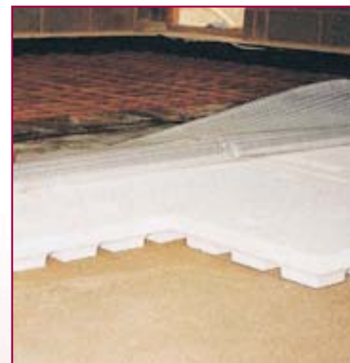
The use of Ventform with its sympathetic surfaces enables the Powerbase membranes to be laid with the minimum of damage.
